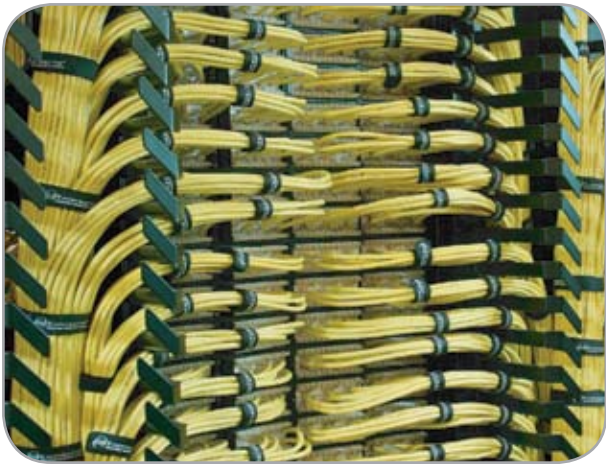
Figure 7. ADC KRONE Cable Racks with Glide Cable Management Systems
